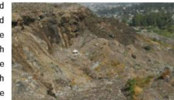
Landfill collapse in Addis Ababa, Ethiopia
