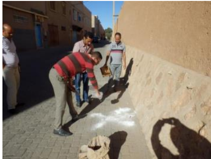
Marking where to install signboards
